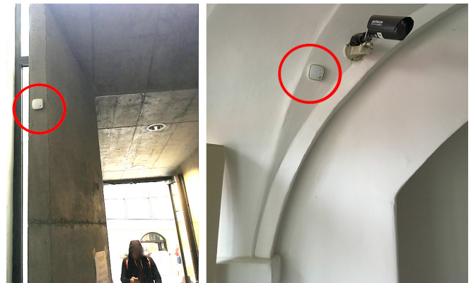
Fig. 2. Beacons installation at the suitable places.
