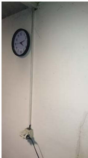
Fig. 5 Illegal socket as a “black” extension of lighting installation
