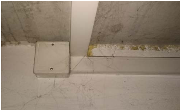
Fig. 4 Modification of lighting installation by screw terminal
